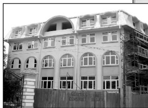
New clinic under construction.
